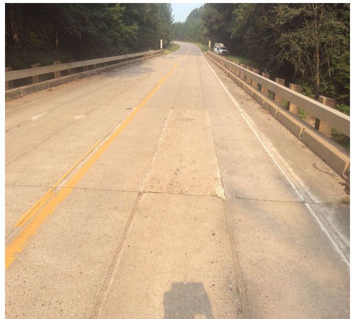
PHOTO 2 Description Some grout missing between channel units near midspan .
