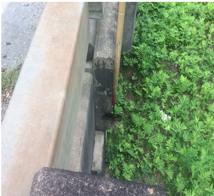
PHOTO 3 Description Bent 12 unit 1 back has moved on cap due to not being bolted and traffic impact.
