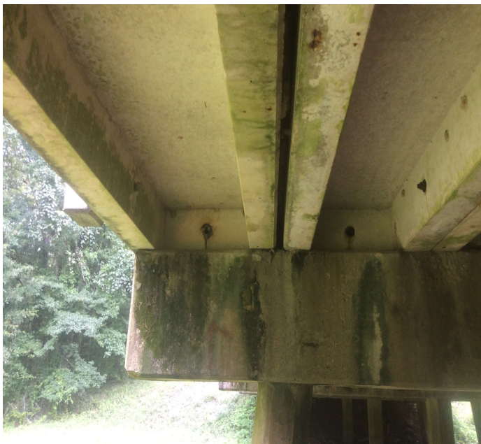
PHOTO 1 Description Span 11 units 1 has separated due to not being bolted and traffic impact.
