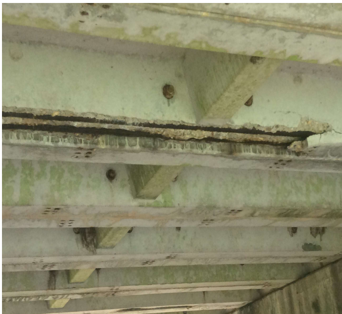
PHOTO 3 Description Span 12 unit 2&3 has large spall with exposed rebar but common on units 7&8.
