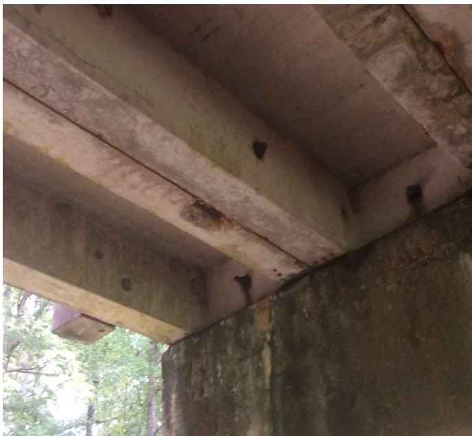
PHOTO 1 Description Small spall with exposed rebar span 6 unit 8.
