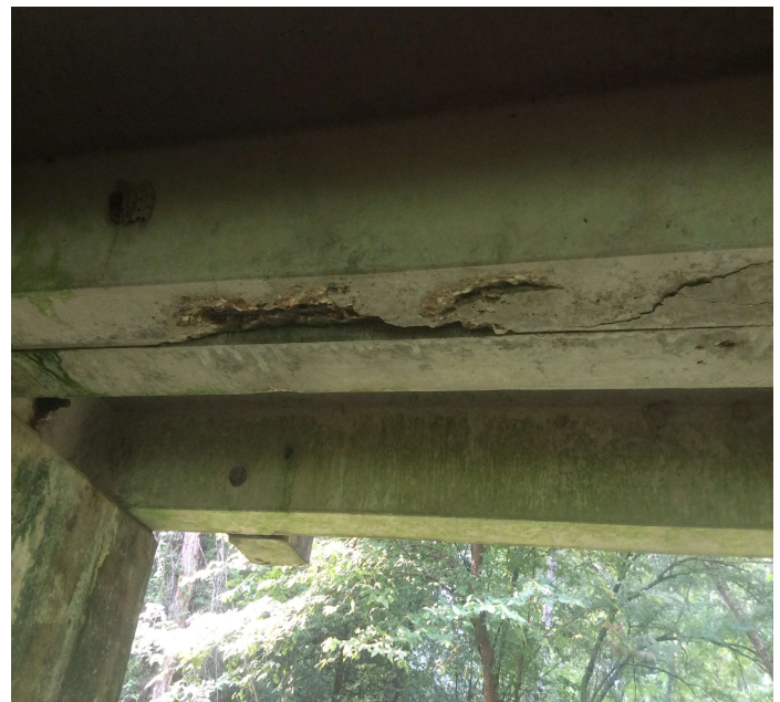
PHOTO 2 Description Span 10 unit 7 has spall with exposed rebar.
