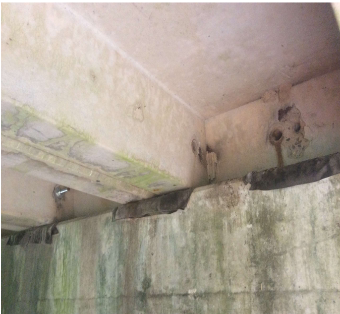
PHOTO 1 Description Span 3 unit 7-8 are not bolted together.
