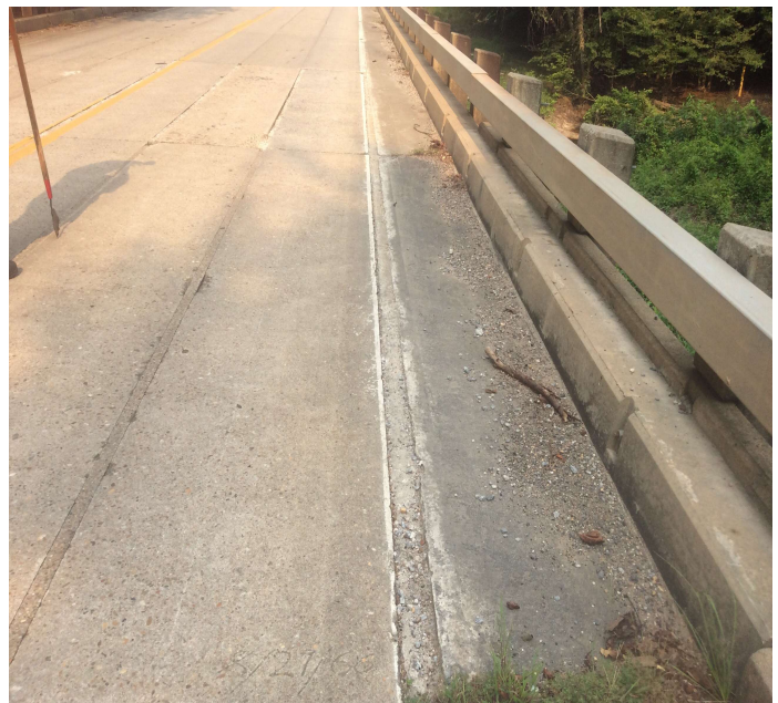
PHOTO 2 Description Grouted keys at span 10 & 11 units 1 & 2 note excessive amount of grout in key due to unit 1 moving from traffic .
